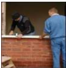
Check Aperture for Defects
